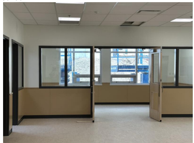
Interior finishing touches are underway.
