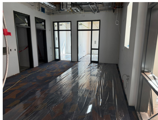
Interior construction progress, April 2026
